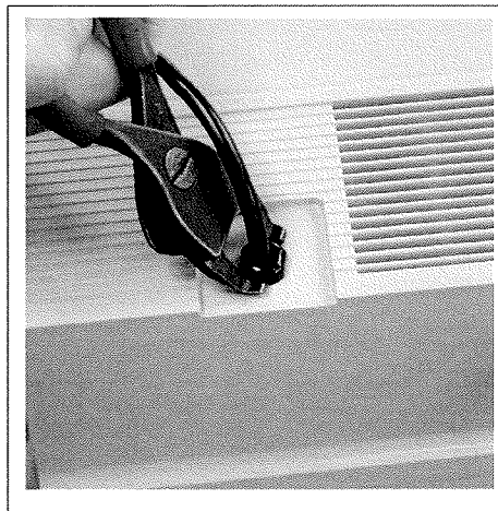
FIGURE 8-4: STRAIN RELIEF REMOVAL
